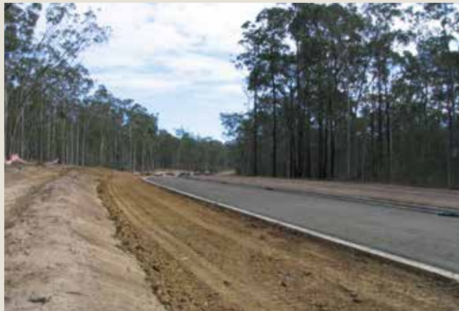
Clearing of Swift Parrot habitat for an industrial estate, Lower Hunter Valley NSW (Mick Roderick).
